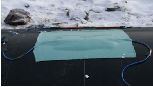
FIGURE 4-STRAIN MONITORING SENSORS INSTALL ON SITE
